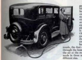
Using the exhaust gas of the automobile to clean the upholstery is the accomplishment of a recently invented device. An aluminum attachment is fastened to the exhaust pipe and the engine is allowed to idle. As the exhaust gas passes through this device suction is created at the inlet hole. Collected by a nozale, the dust and dirt are drawn
